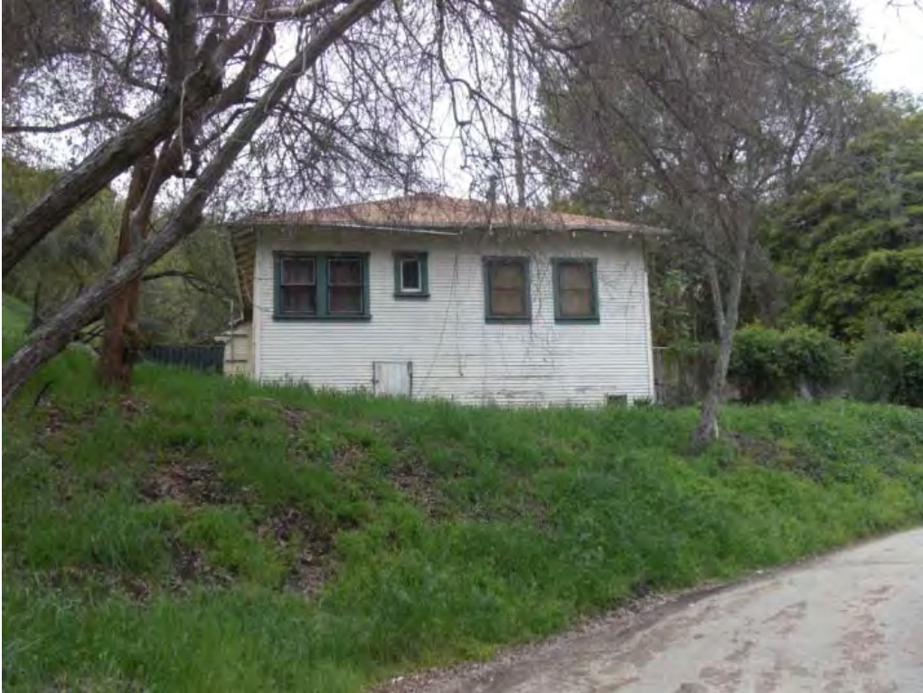
5. 3705 Coldwater Canyon north elevation
