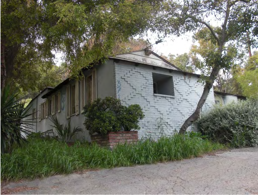
7. 3719 Coldwater Canyon south and east elevations
