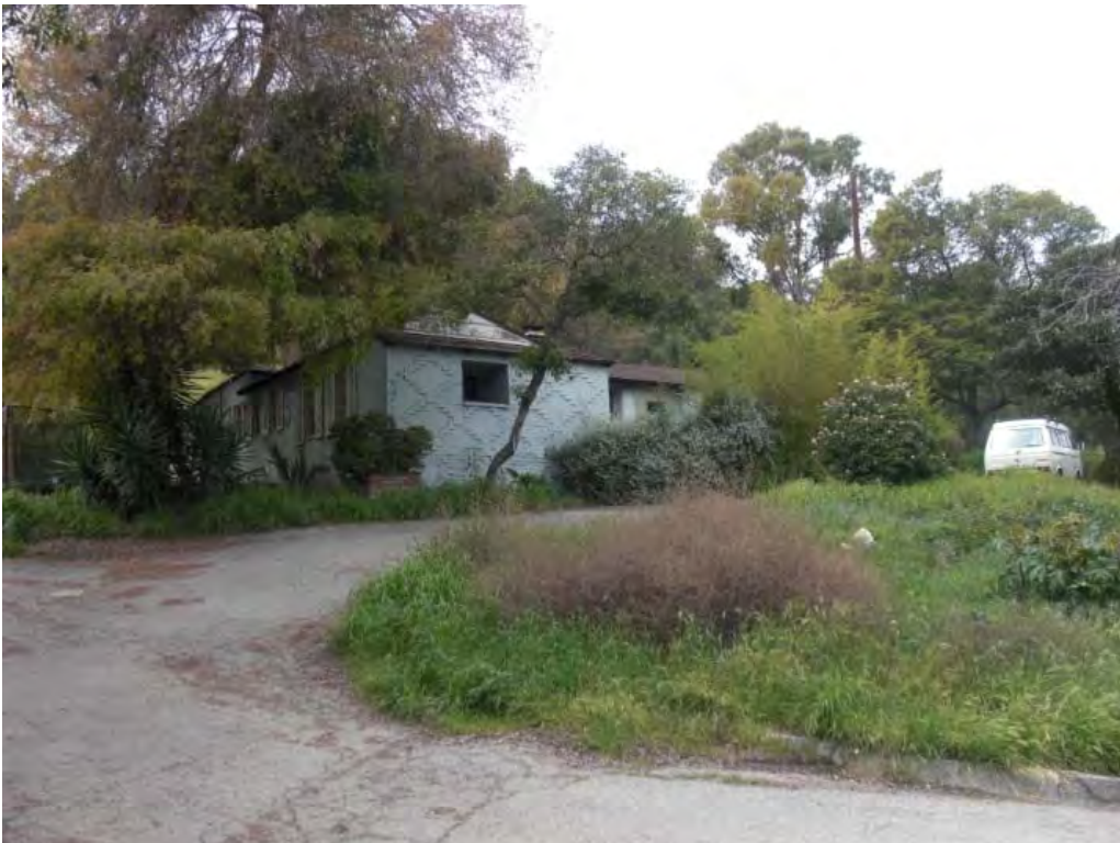
6. 3719 Coldwater Canyon street façade
